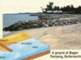
The deposition of sediments on one side of a groyne causes the unprotected side of the coast to be deprived of these sediments and to be eroded by waves.
