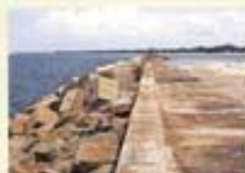
A breakwater with sediments inside the harbour at Chendering, Terengganu.
