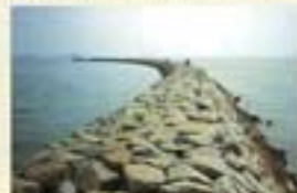
A structural jetty made of rocks at Melaka.
